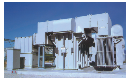
Fig. 5 All-film Power Capacitor Contained in Dead-tank
