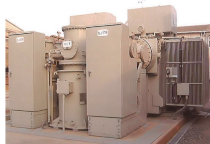
Fig. 8 AE-type Compact GIS
