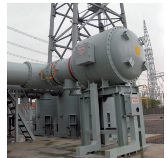
Fig. 7 Gas Insulated Voltage Transformer
