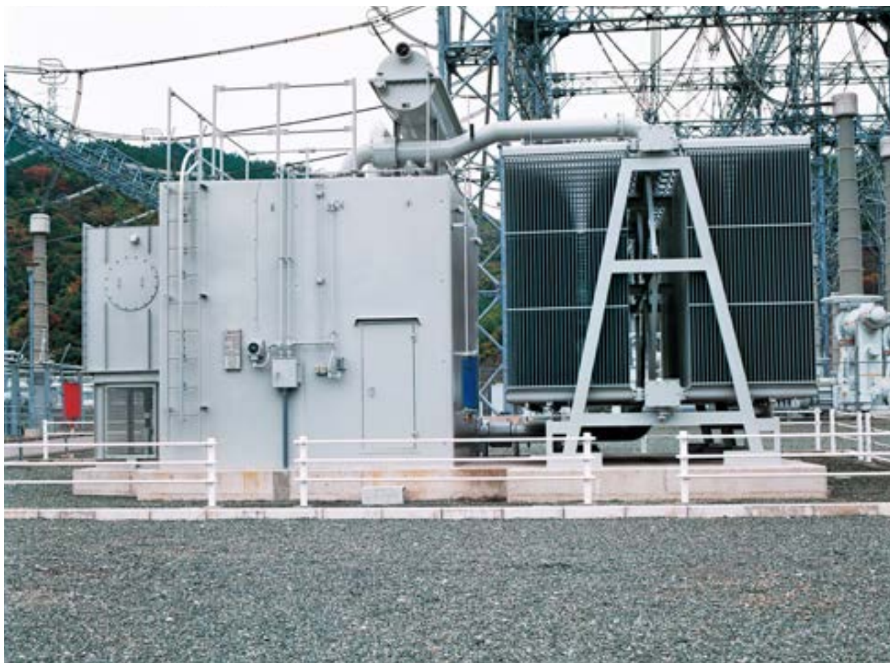
3φ 60Hz 60kV 100,000kVA (60ホン)
