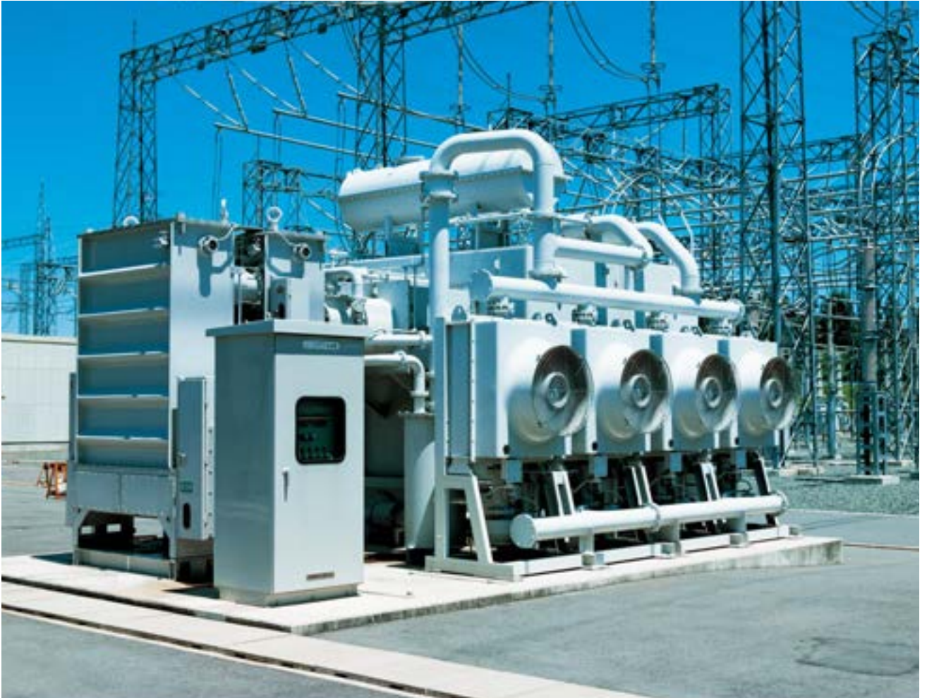
3φ 60Hz 66.5kV 100,000kVA(65ホン)
