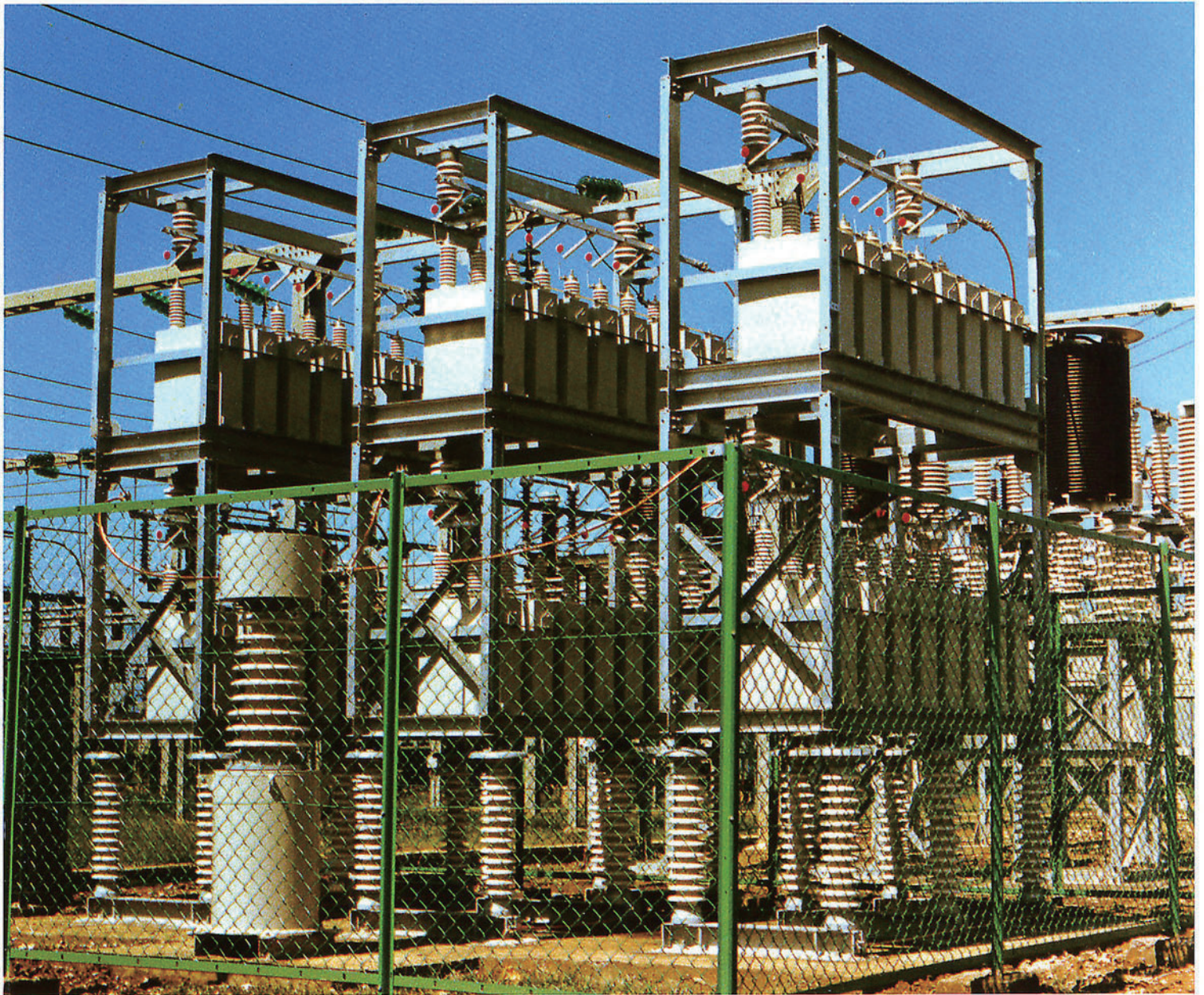
Shunt capacitor bank 66 kV 3 \phi 50 Hz 10 Mvar
