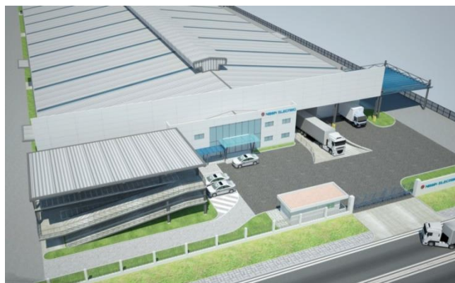
Image of renovated Plant 1
