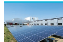
Captive Consumption Photovoltaic System
