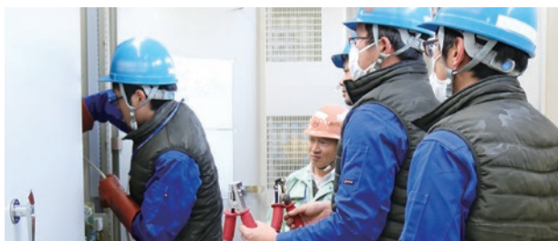
Customers learning how to shut down and restore substation equipment using an actual machine
