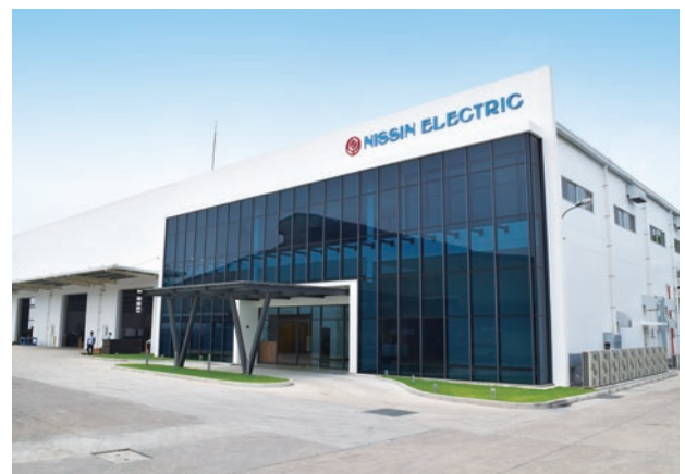
External view of Factory 2 at Nissin Electric Vietnam
