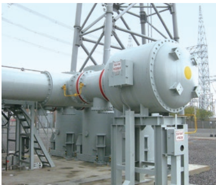
1,000kV Gas Insulated Voltage Transformer (UHV VT)
