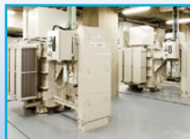
22/33kV Spot Network Substation Equipment
