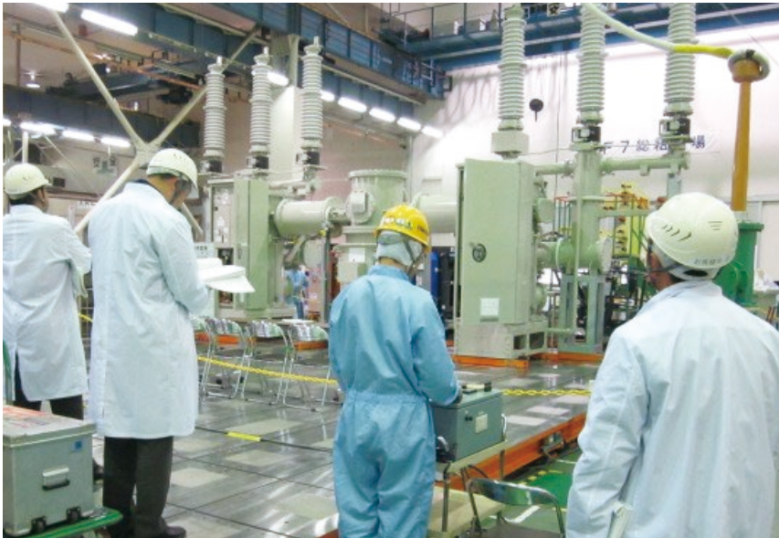
Pre-shipment onsite inspections of our products by our customers
