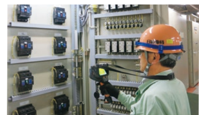
On line inspection
