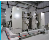
66/77kV Gas Insulated Switchgear (indoor type)
