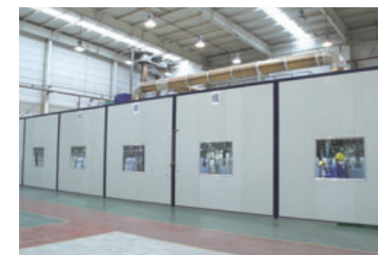
Painting line with the addition of an active carbon air collector
