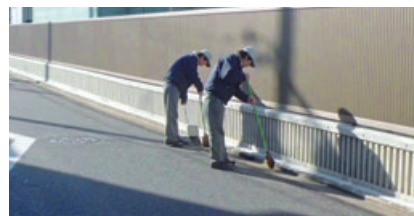
Clean-up activities around the works
